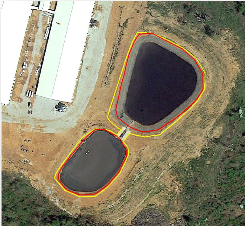
Figure 12. Yellow outer boundary denotes the drainage area (59,457 ft 2 ) into the holding ponds. The red inner boundary denotes area of the top of the free board for holding Pond 1 (16,999 ft 2 ) and Pond 2 (34,618 ft 2 ).
