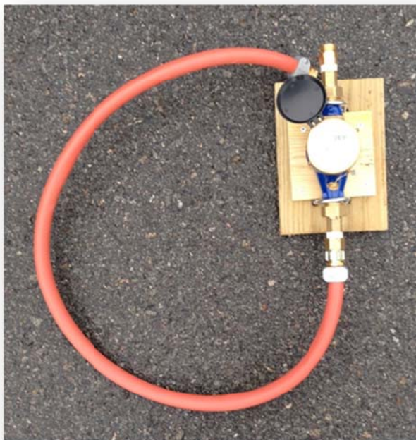
Figure 8. One of the standard water meters with hose adapters and mounting base installed to measure water use during pressure washing to clean animal pens.
