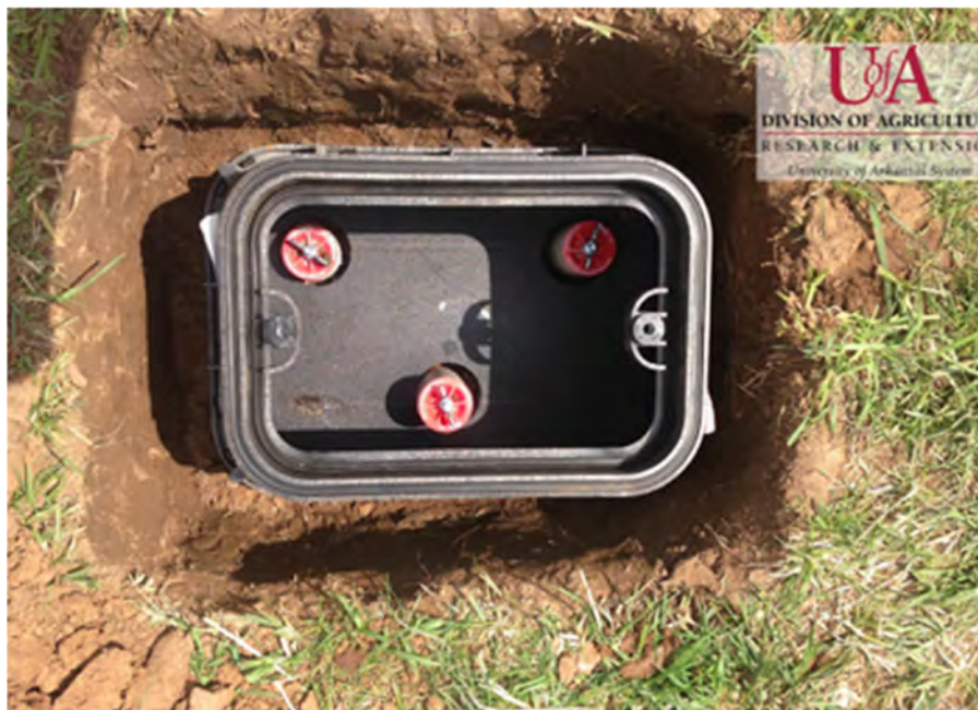
Figure 4. Construction of belowground piezometer.
